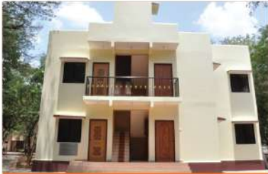
GRFG-Building IITM Chennai
