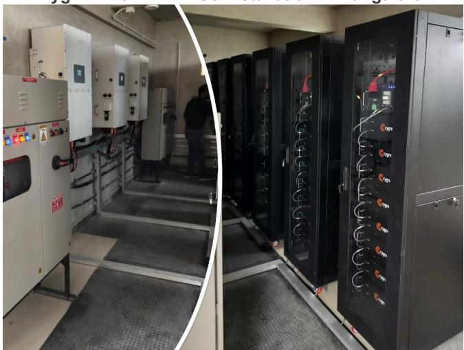
Cygni Energy successfully deployed a 240 kWh Battery Energy Storage System (BESS) at a reputed educational institute in Bangalore, designed to enable seamless off-grid operation and reliable backup support. During daytime, the solar energy simultaneously powers the campus load and charges the battery, ensuring that once solar production tapers off, the BESS continues supplying uninterrupted power—resulting in minimal to zero grid dependency.
